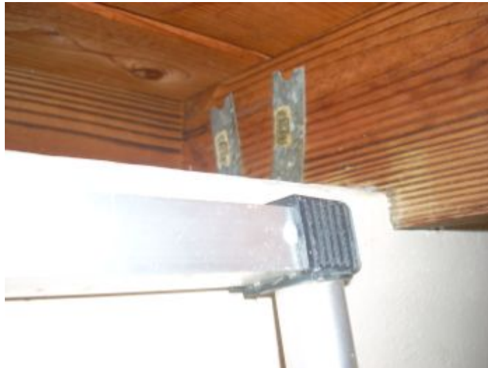
Example of double straps on rafters
